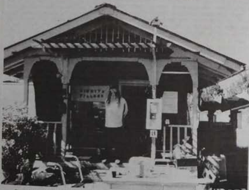
Tim in front of Dignity's Community House, the first structure they built, a strawbale house.
