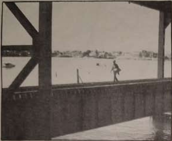
Portsmouth Harbor rail bridge,
